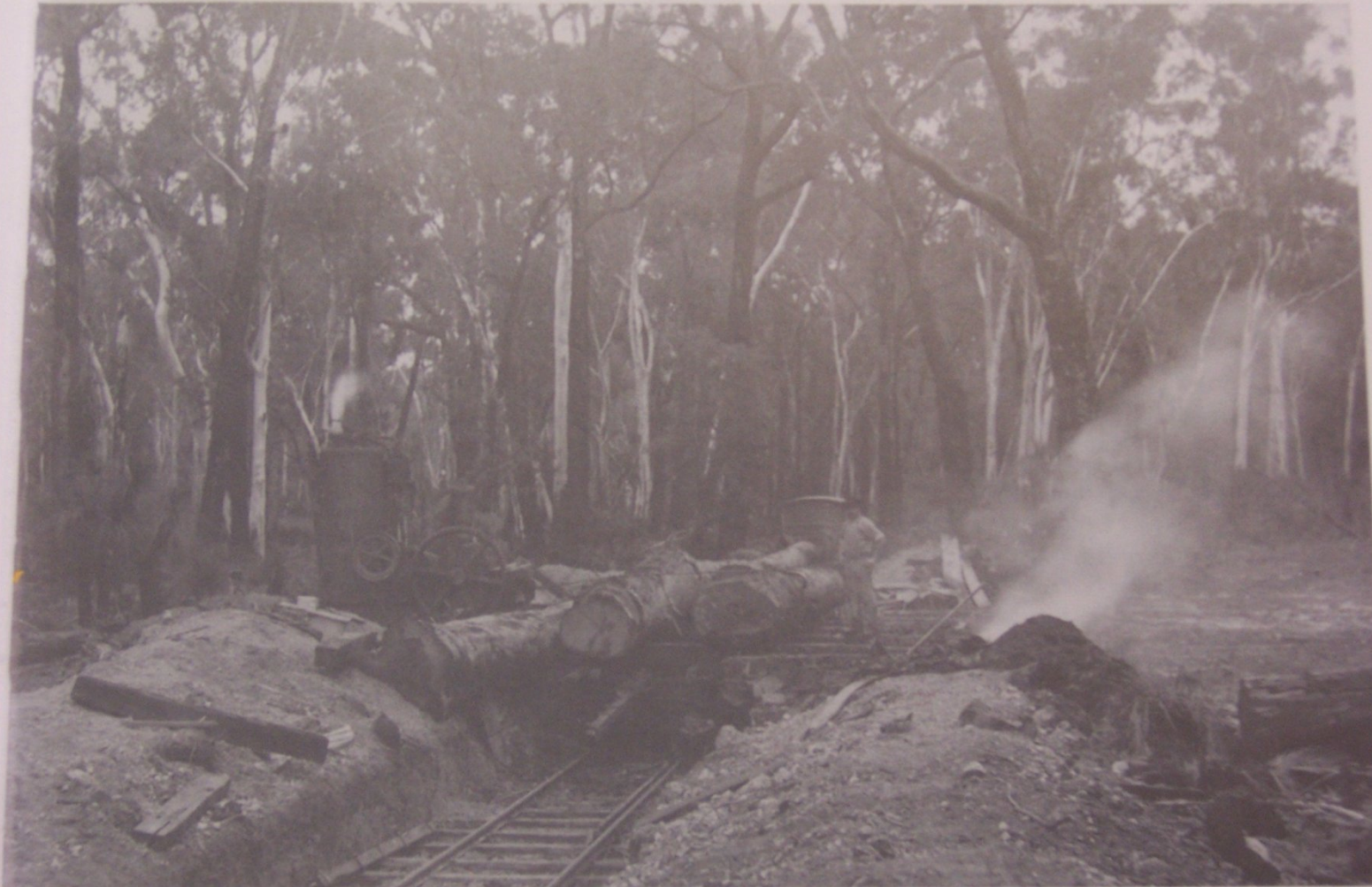
A steam winch rolling logs onto a 'set' at a typical bush landing.
